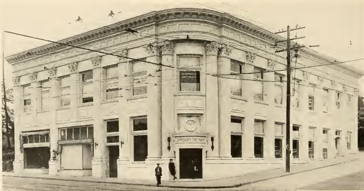
UNIVERSITY STATE BANK BUILDING, SEATTLE, WASH.
